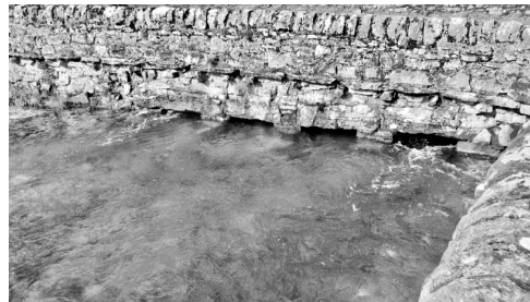
Photo 3 Road bridge culvert, stone slabs spanning over stone piers, needs cleaning out, a grade II listed building
