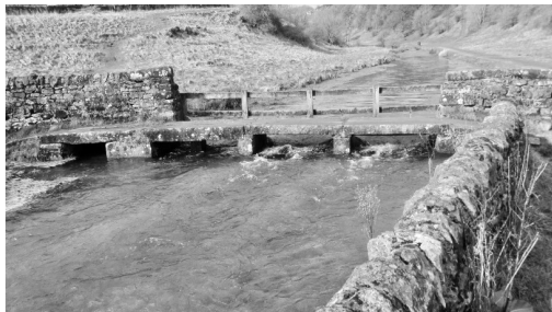
Photo 2: Clapper footbridge at Stoneyside, stone slabs spanning over stone piers, a grade II listed building
