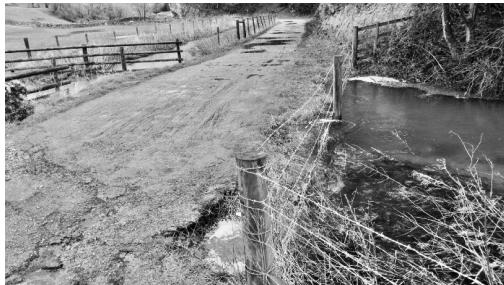
Photo 1: Coach Road, 1950's blocked culvert with concrete slab over, River Bradford entering from the right at road level
